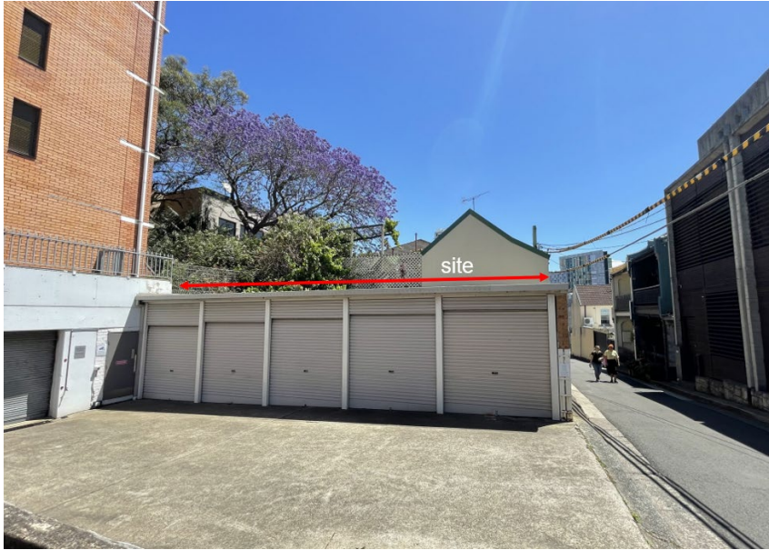
east elevation viewed from Wells Street
