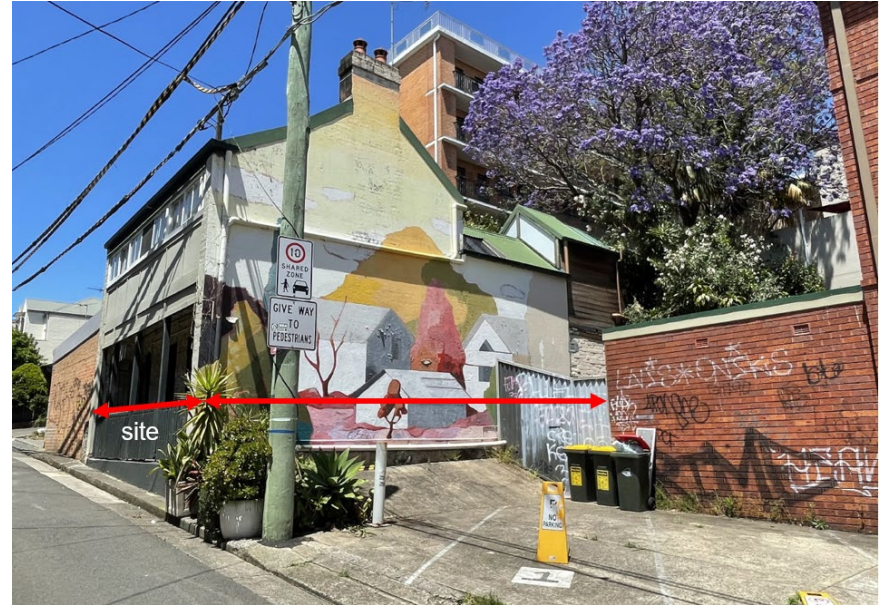
west elevation viewed from Wells Street - showing existing rear addition
